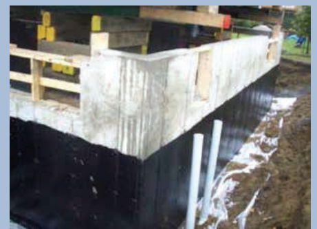
Correct installation of chimney (solid PVC pipe) showing stand-off from the wall and placement of plastic barrier on top of the gravel - ready for back-fill.
