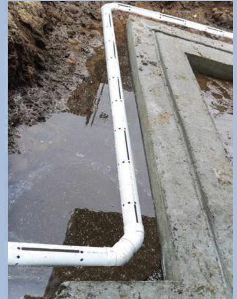
Pipe with 7-hole pattern installed along a footing with the print line facing upward.
